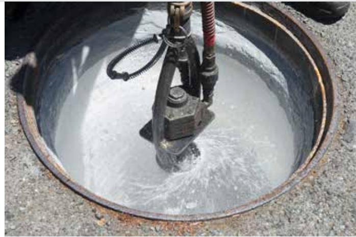
LEFT: Jesus Uriarte lowers a modified Madewell Spin Caster into a manhole during a rehabilitation project. BELOW TOP: The Spin Caster sprays an even coat of composite liner around the interior of the manhole. BELOW BOTTOM: The rehabilitated manhole lined with Mainstay composite material.
