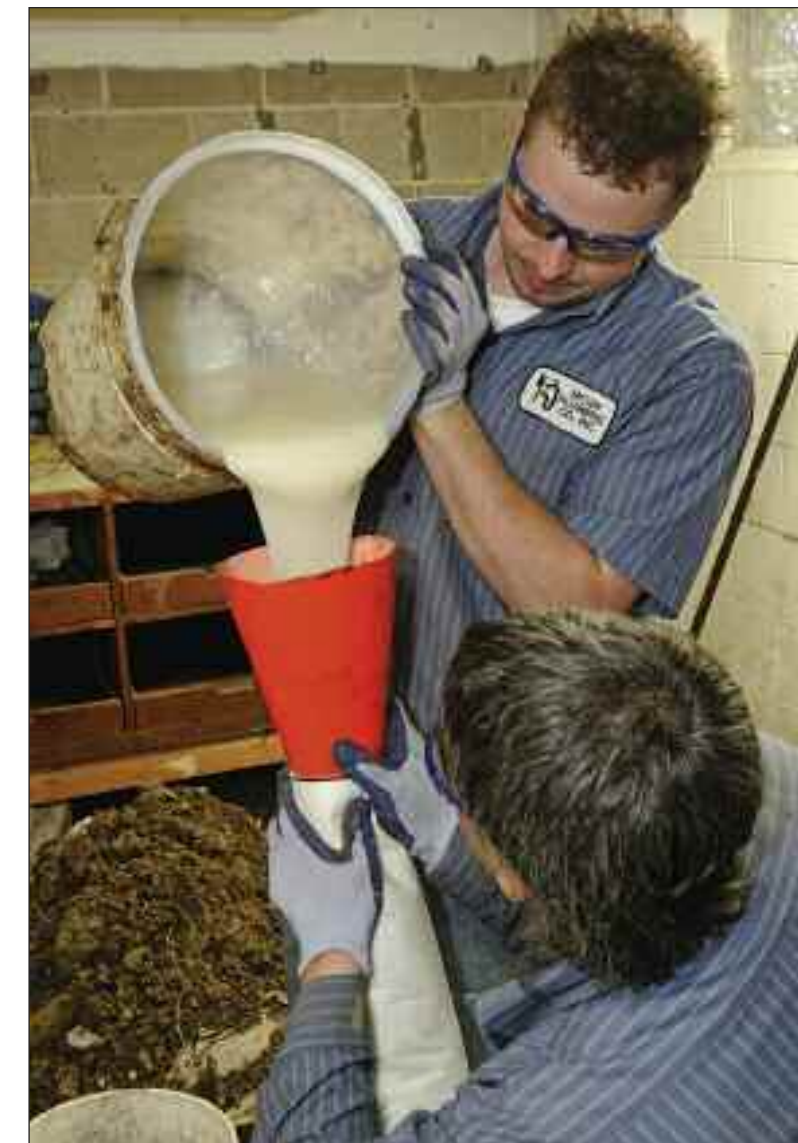
Above, Michael McVay, Mike Heilmann and Brad Plata clean a line with a RIDGID KJ-3000 jetter and a nozzle from Arthur Products. Right, Brad Plata introduces Perma-Liner resin into liner held by Michael McVay.
