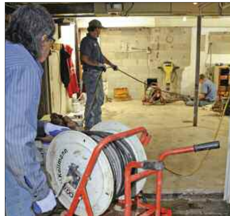
Above, Michael McVay, Mike Heilmann and Brad Plata clean a line with a RIDGID KJ-3000 jetter and a nozzle from Arthur Products. Right, Brad Plata introduces Perma-Liner resin into liner held by Michael McVay.
