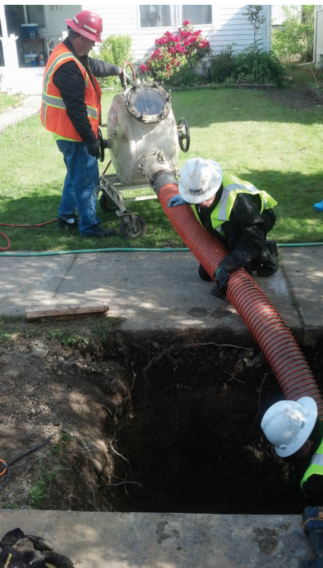
From left, Project Manager Mike Wasmund, CIPP tech Thomas Tyron and Nick Patrick feed a liner into a residential sewer lateral.
