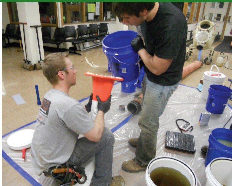
John Thomas from SLB Pipe Solutions prepares to pour the hot resin mixture into the 6-inch liner while SLB Pipe Solutions co-owner Joel Langebartels steadies the receptacle. (Photos courtesy of SLB Pipe Solutions)
