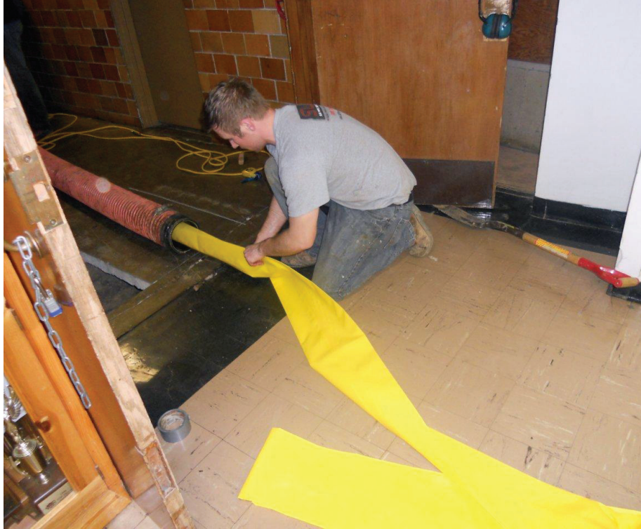
Joel Langebartels helps feed the calibration tube into the inversion tube on the job site at Franklin High School in Franklin, Ill.
