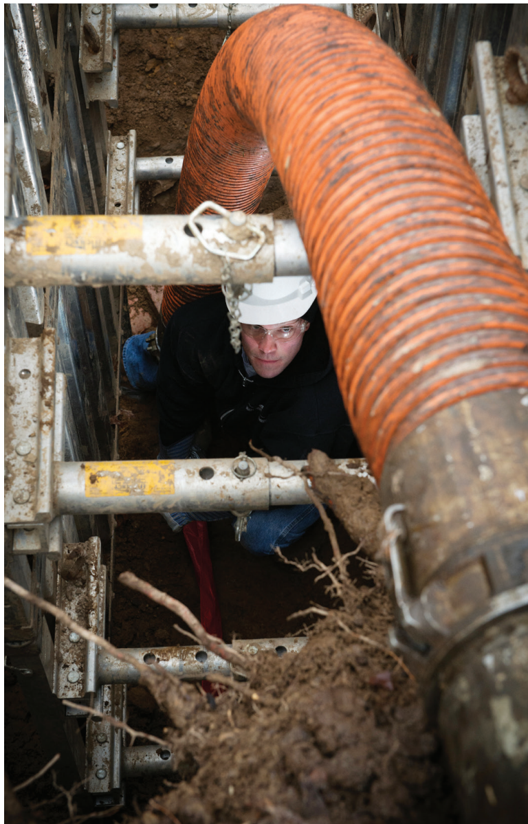
Matt Mertz, owner of Matt Mertz Plumbing, stands in a shoring box while installing a lateral liner for a residential customer.
