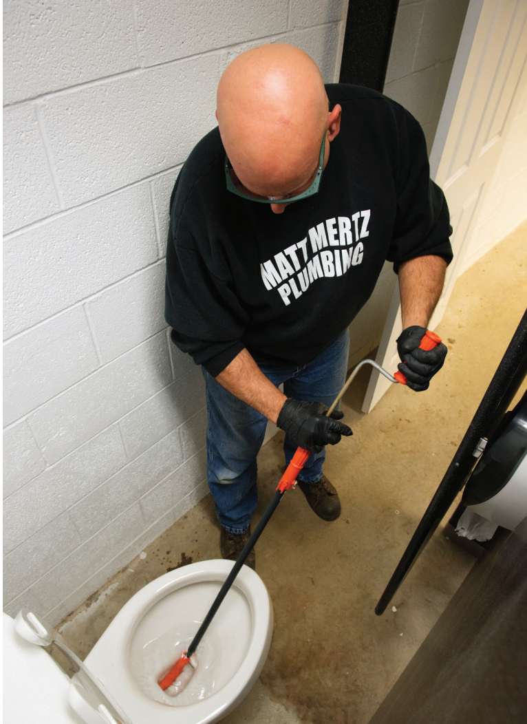
Master plumber Phil Arena uses a closet auger to open a clogged toilet at a private residence.
