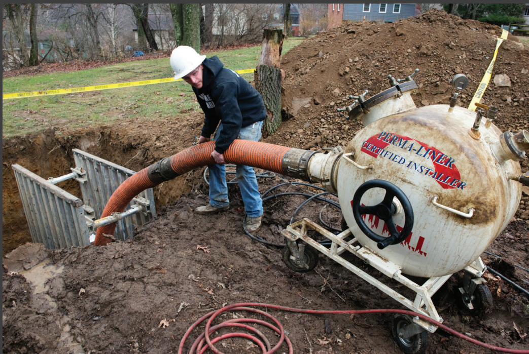
Dylan Belfiore guides the Perma-Lateral inversion unit at the entry pit on a lateral relining job.
